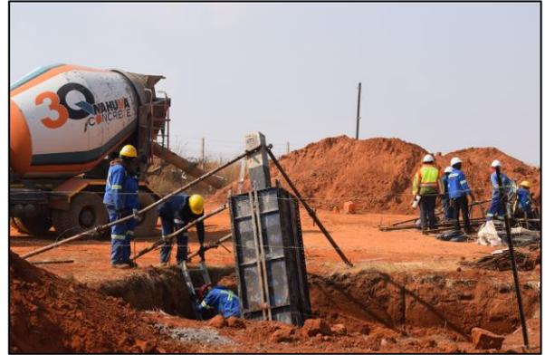
Figure 3: Cement filling for tower foundation
