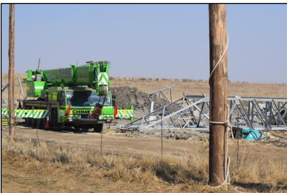
Figure 6: Tower ready for Assembly
